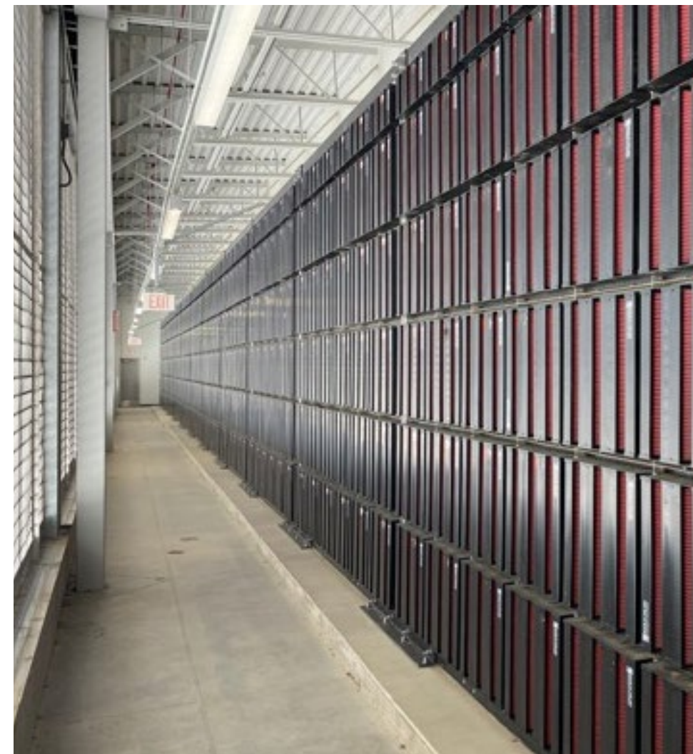
In 2023, we fully switched to reusable air filters to reduce waste sources — like packaging materials and commonly used equipment.
